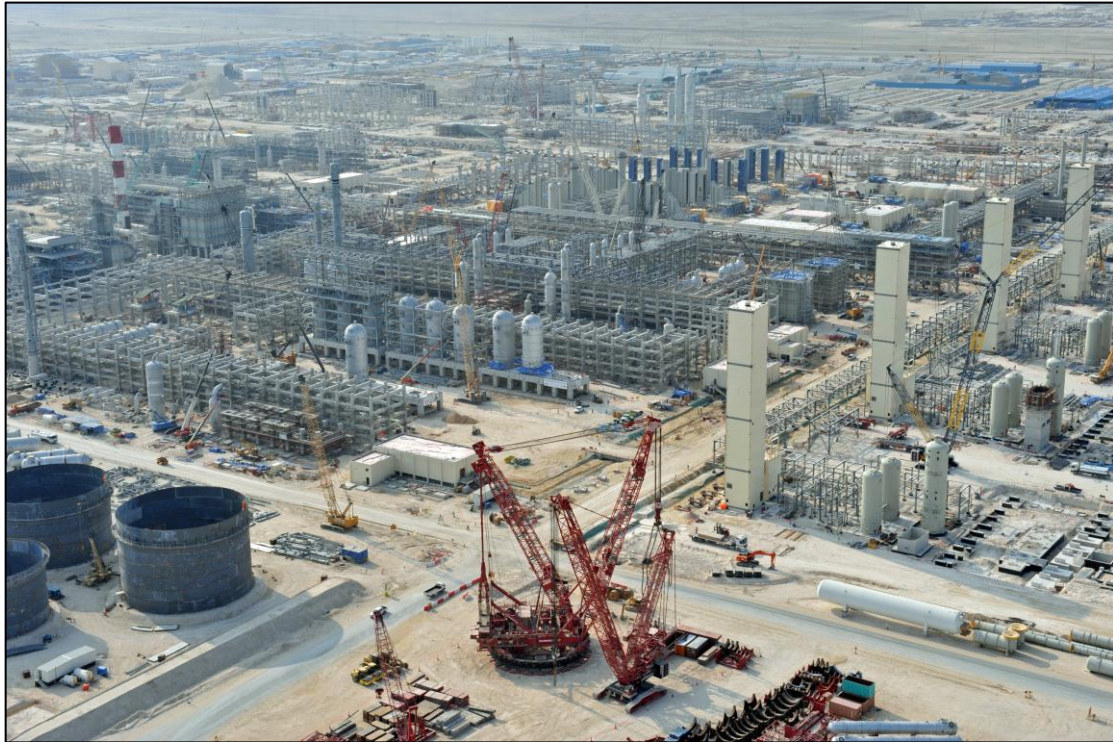
On-going construction at the Full Field Development project in Abu Dhabi
